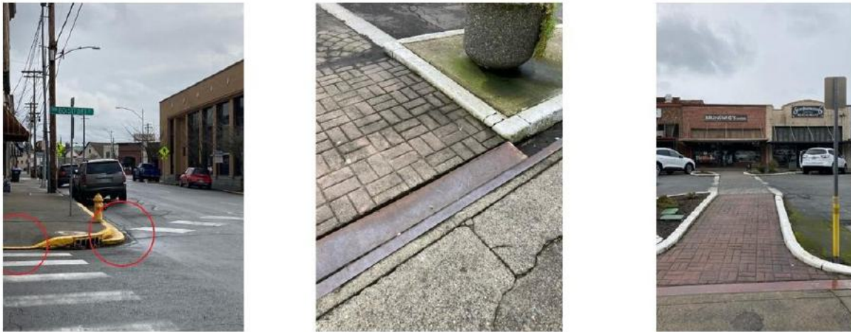
Figure 9: Sidewalk Conditions (clockwise): Material, level differences and lack of accessible ramps.
