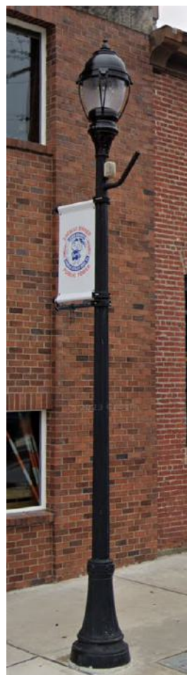
Existing light fixture on NW Pacific Ave adjacent to project area; Stresscrete Group King Luminaire with Hapco York Series Pedestrian Pole
